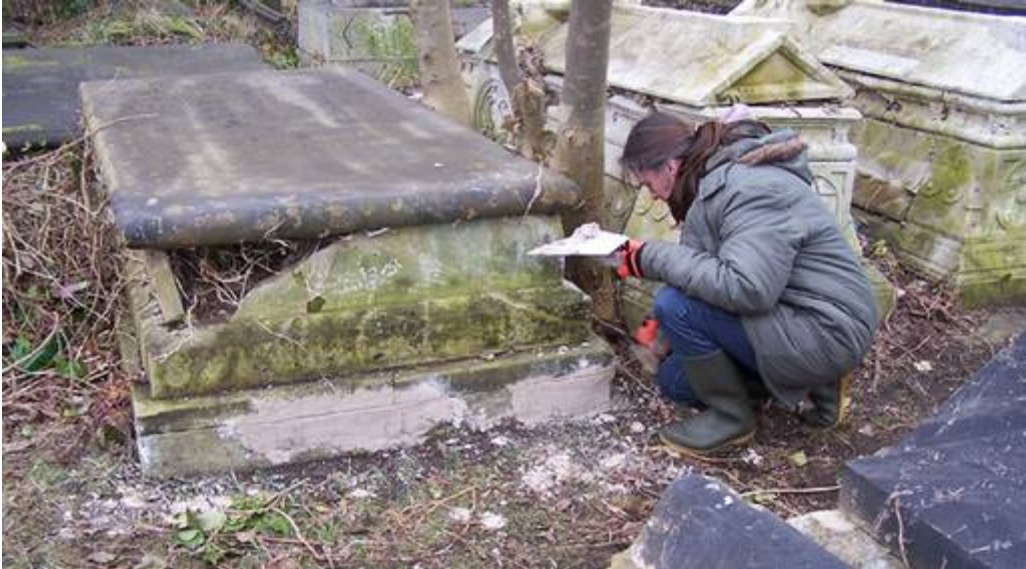
Cathy learning to apply lime mortar, February 2013
