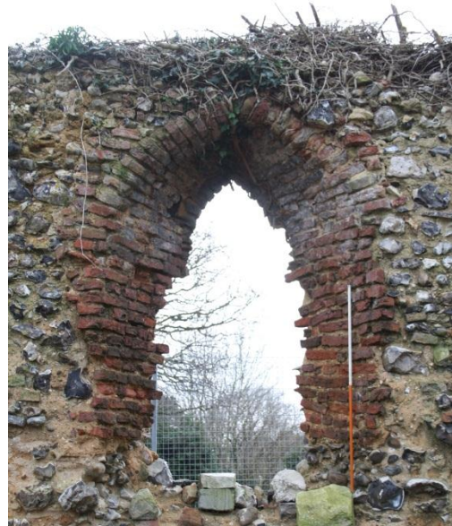
The head of this brick lancet can be seen in this southern wall window although the jambs are much eroded
