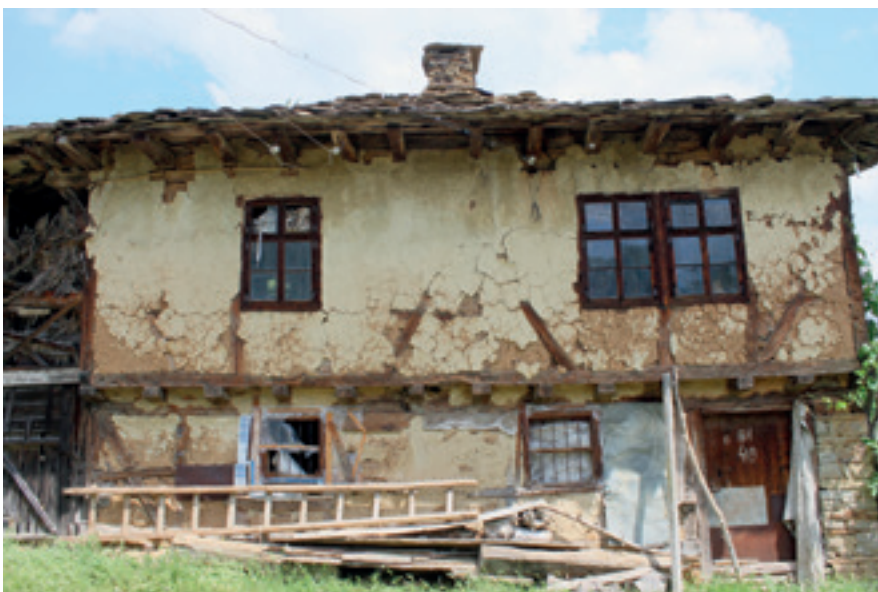
A traditional dwelling in the village of Karpachevo with typical construction of stone plinth, timber frame with adobe bricks and low-pitched roof bearing unsecured stone slates
