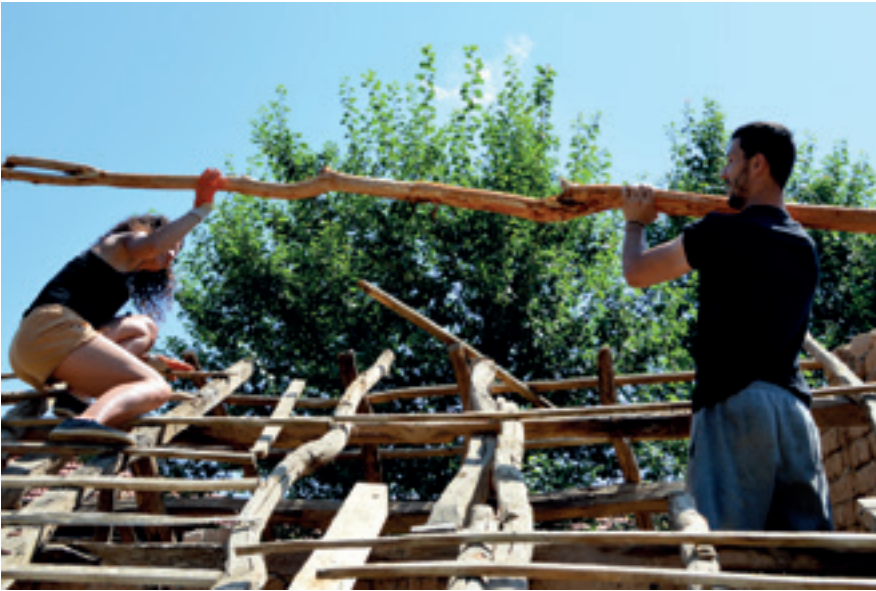
Volunteers carry out roof repairs
